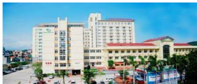
Fig 1 - Bai Chay Hospital development
