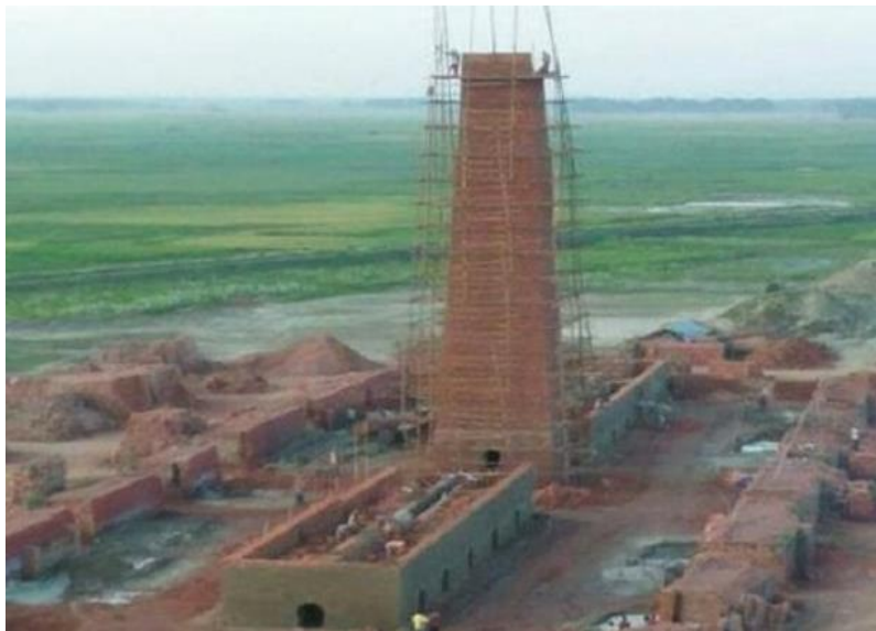
Figure 1: High draught Zigzag kiln. (Source: The Express Tribune)
