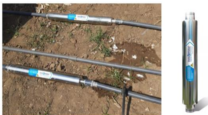
Fig.2. Installing magnetic devices on main lines for network irrigation system.
